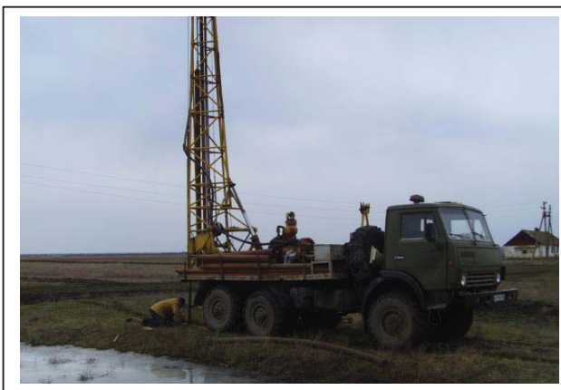
Figure 12. The drilling equipment
